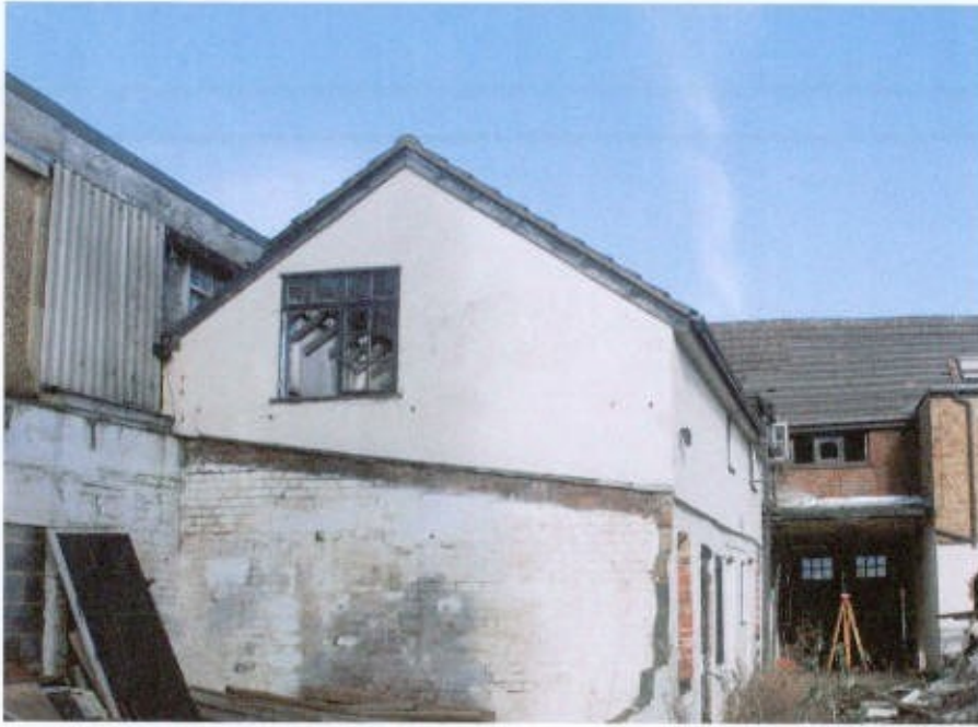
4.1.3 Rear of the front building
