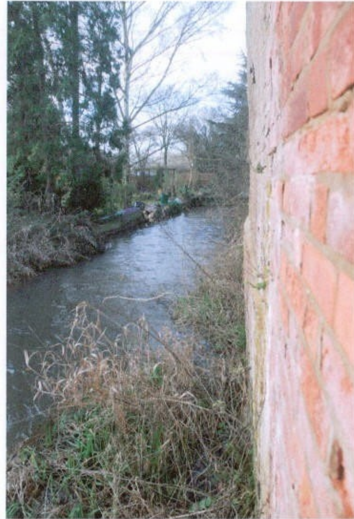
4.1.4 Existing building on the river bank
