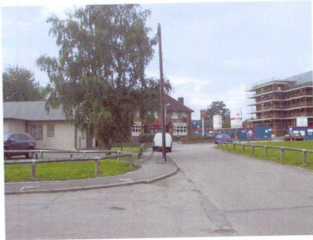
View of the site looking west along School Mead. The site and existing Hall are to the left of the picture. The Breakspeare Public House is in the centre. The local shopping facilities (under construction) in the background and public open space in the foreground are to the right.
