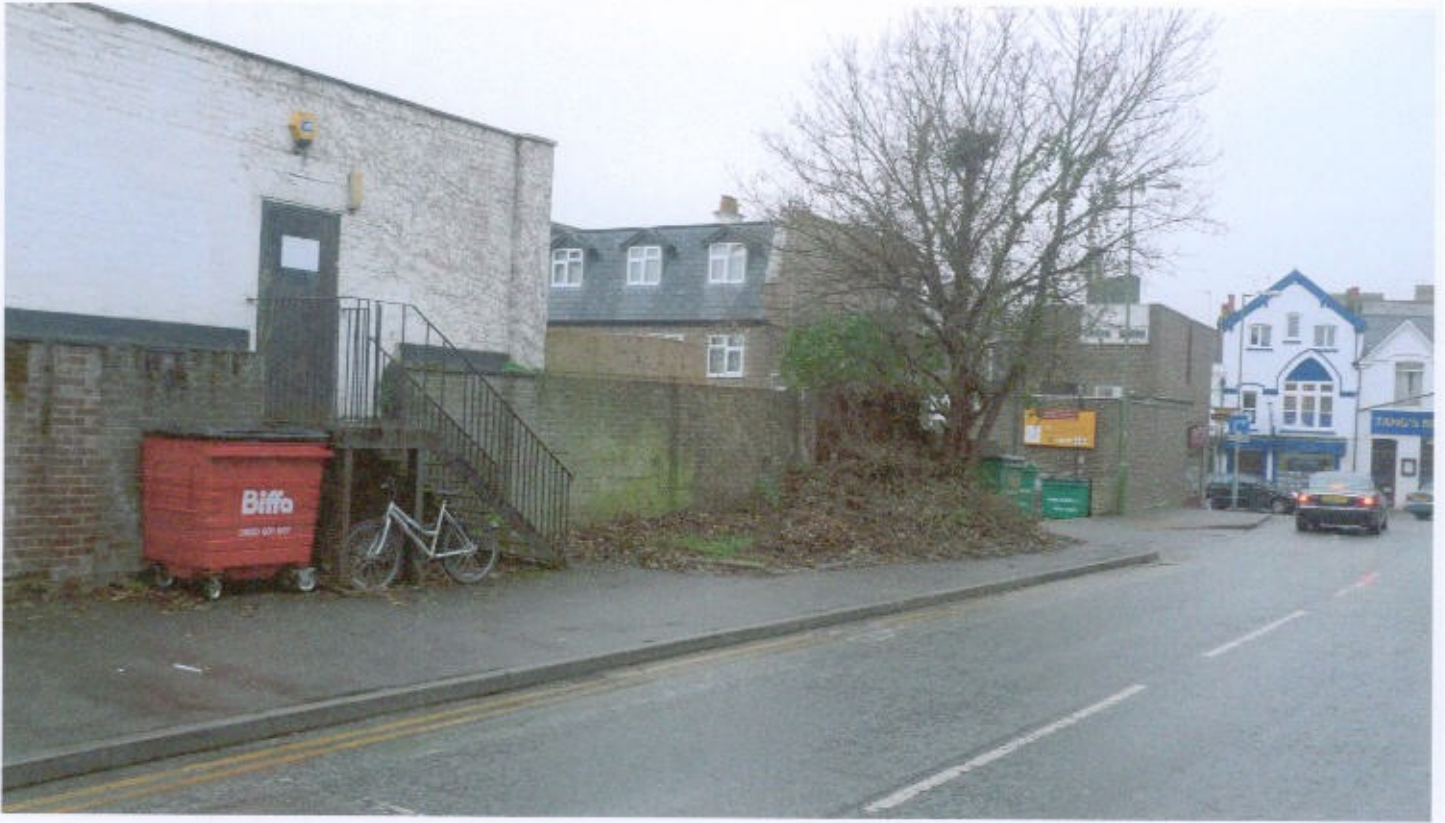
View of rear of No's 4 & 6 Station Road from Northway
