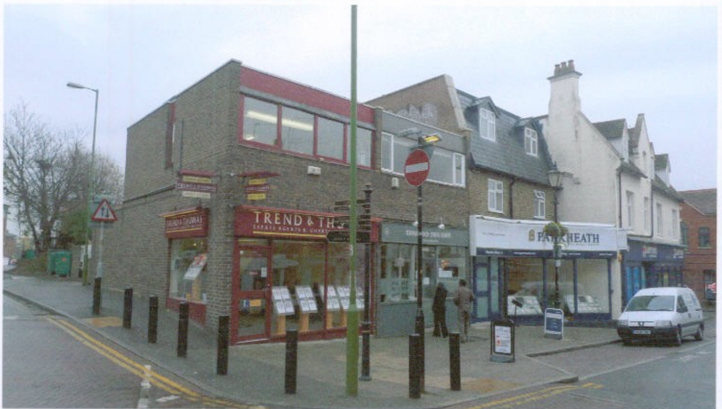
View of No's 4 & 6 Station Road from junction with Northway
