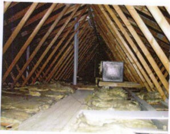
Photograph 12: Southern long tall loft
